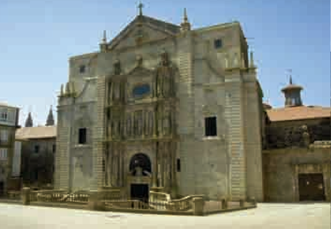
Church of San Martín Pinario façade
